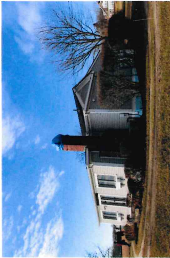
EXISTING BUILDING (VIEW FROM NE)
