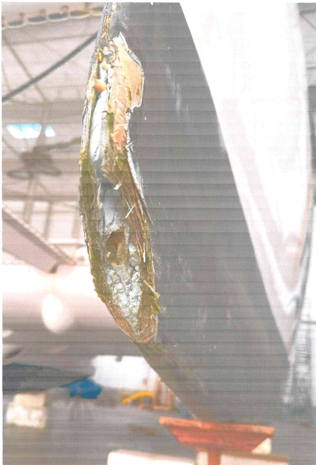
Damage at Bow – at and below waterline
