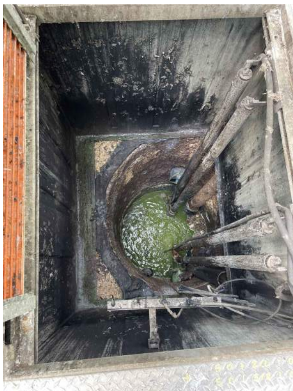
LIFT STATION 8 WET WELL (INTERIOR)
