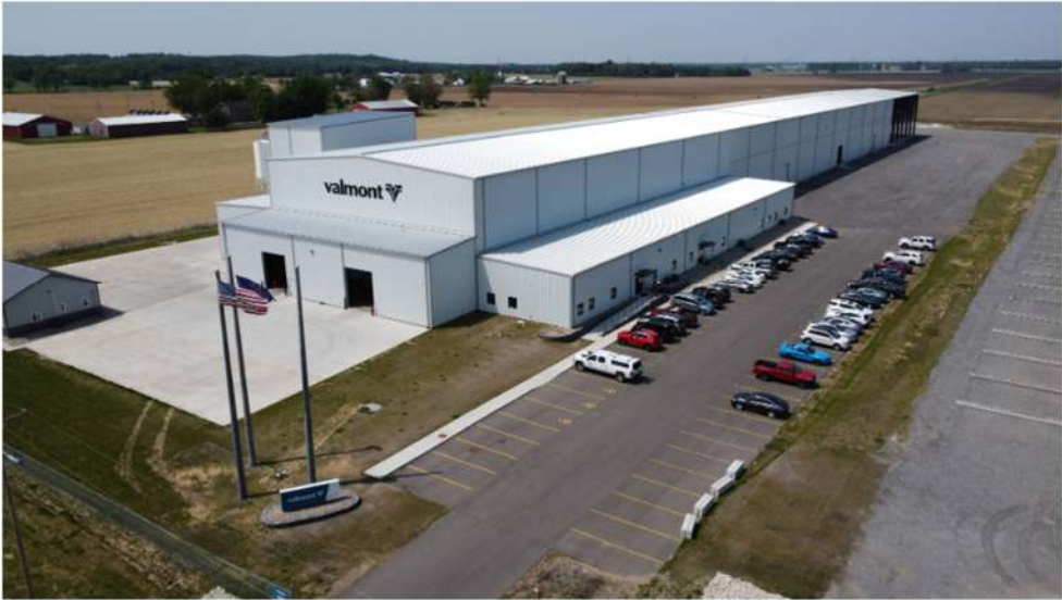
Valmont Industries Inc, Bristol facility
