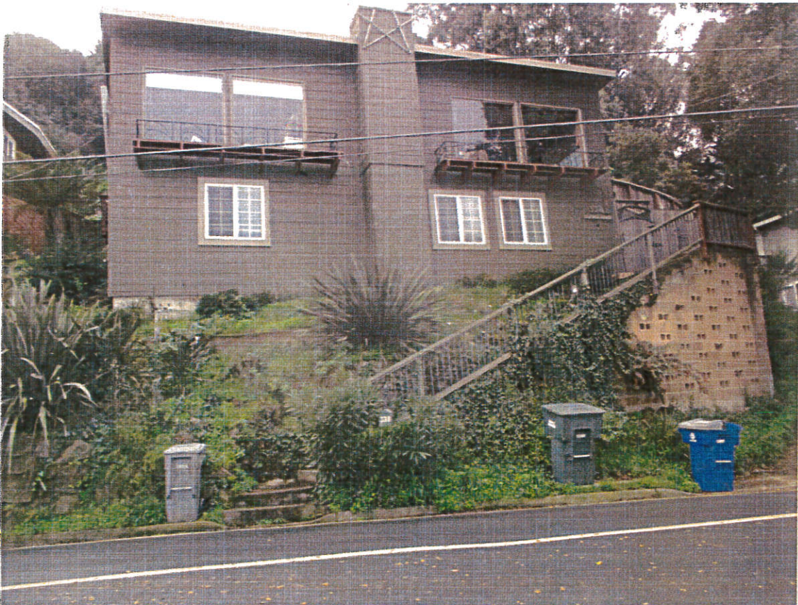
Photo 1: View of the front of the residence from Kings Road. The garage addition is planned on the right side of the residence (on the right side of the photo).
