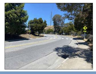
The Crocker Park Recreational Trail crosses South Hill Drive at the apex of a curve. There is an existing marked crosswalk located approximately 80 feet north of the trail location. The crossing includes double sided pedestrian crossing signs with RRFB warning lights and advance pedestrian warning signs with RRFB warning lights in advance of the crossing in each direction. There are no signs which direct trail users to the marked crosswalk.
