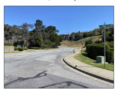
An existing midblock crossing is provided with pedestrian warning signs on each side of the crossing. Existing speed limits are 30 mph north of the crossing and 40 mph south of the crossing. Shoulder buffered striping is provided on the west side.
