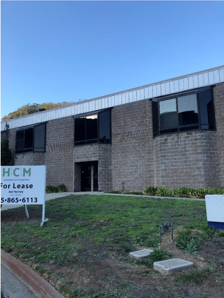
View of the front yard from W. Hill Pl. looking north.
