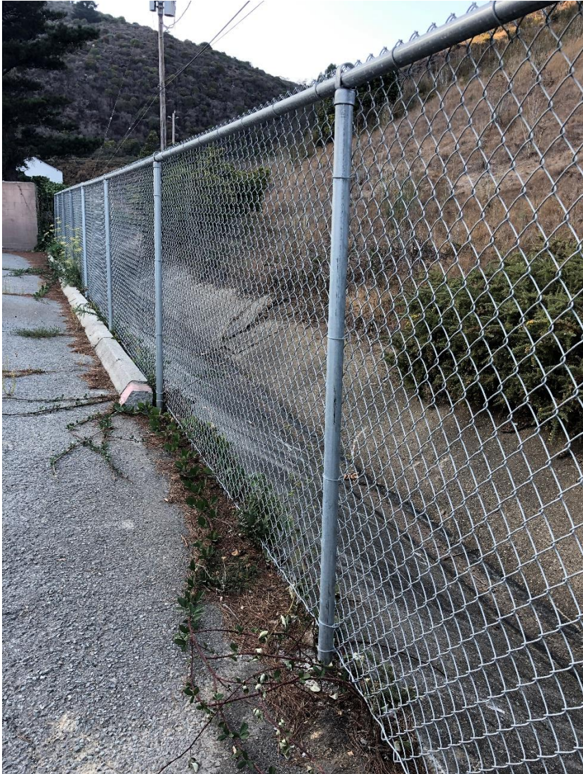
View of concrete v-ditch within City easement.
