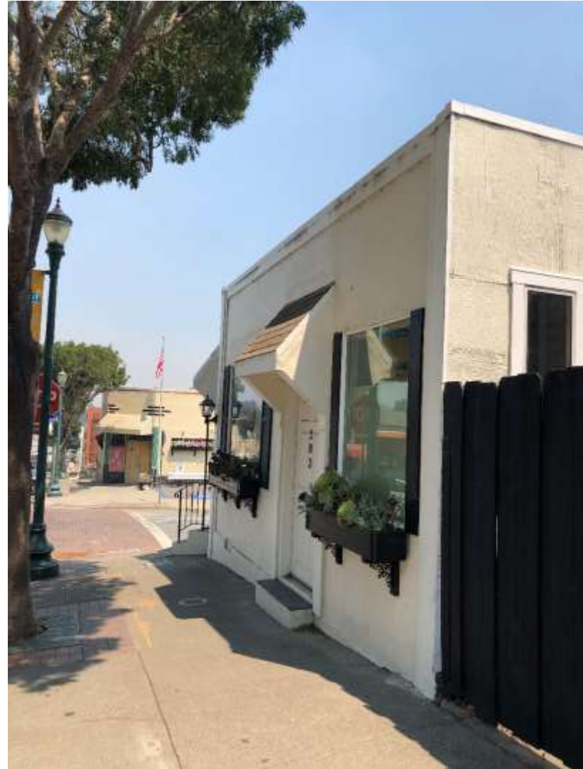
View of 201-203 Visitacion Ave. (north of subject property)
