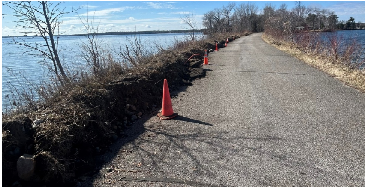
Figure 2: Shoreview Lane Existing Conditions - South Facing
