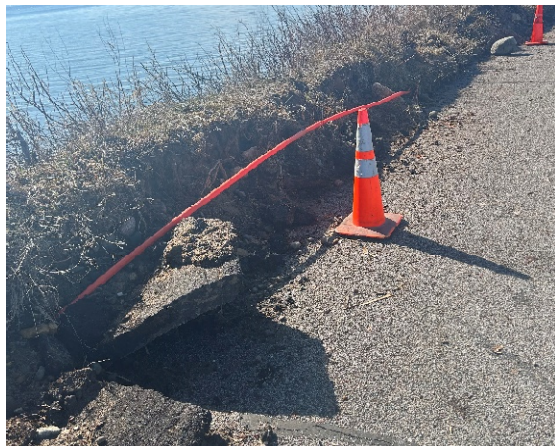
Figure 3: Exposed Utility
