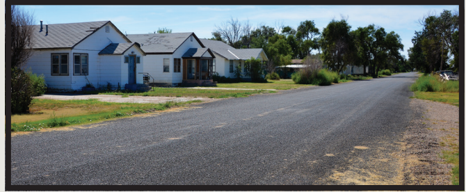
Street in Walsh, Colorado, that was repaired doing Full-Depth Reclamation with their Asphalt Zipper® and then chip-sealed.
