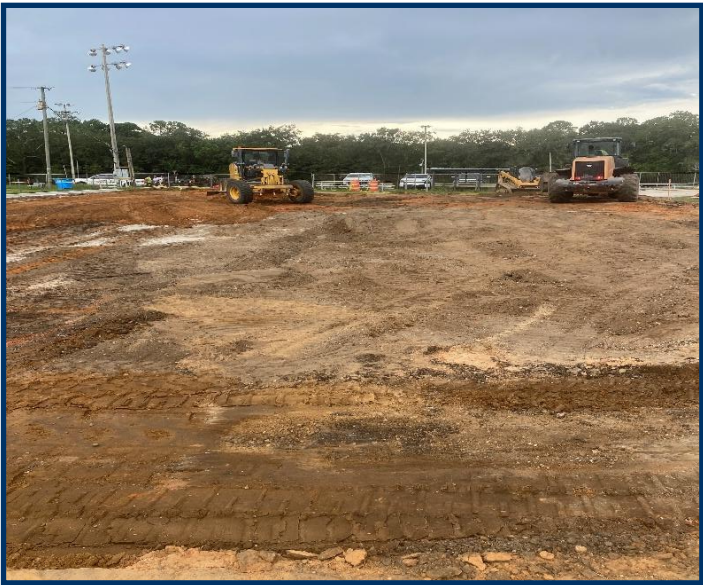
Bonifay Memorial Field Drainage Improvements Contractor removing existing dirt and grading Southside Parking Area on Veterans Blvd.
