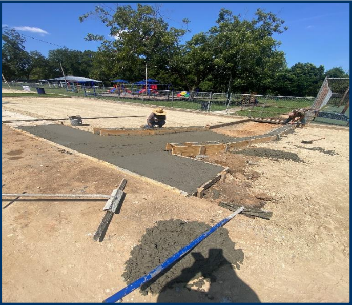
Bonifay Memorial Field Drainage Improvements Contractor installed and finished NS concrete for flume and curb at Sta. 28+20 LT side.
