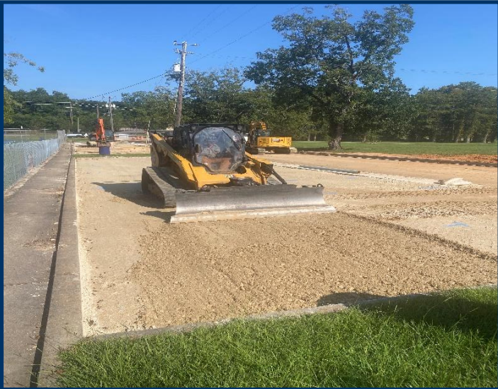
Bonifay Memorial Field Drainage Improvements Contractor installed Optional Base Material in parking bay on Northside of Veterans Blvd.
