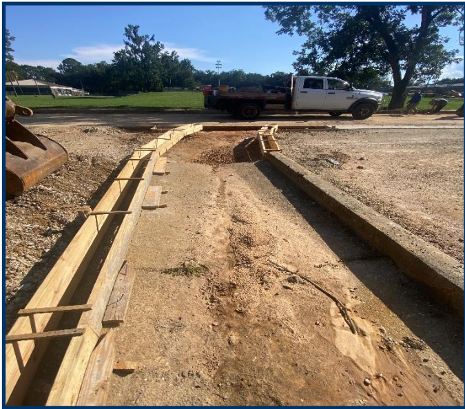
Bonifay Memorial Field Drainage Improvements built form for flume and curb at Sta. 28+20 LT side.
