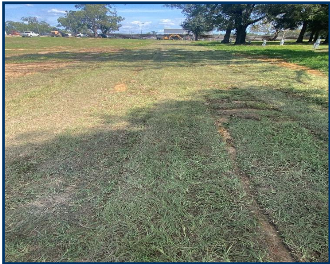
Bonifay Memorial Field Drainage Improvements Contractor installed Performance Turf Sod in field between Depot St. and McGee St.
