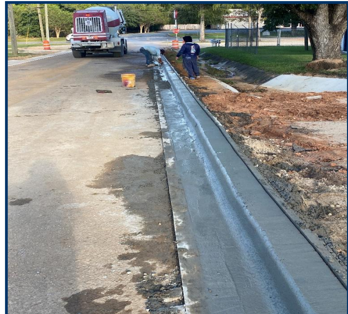
Bonifay Memorial Field Drainage Improvements Subcontractor installed NS concrete and finished curb and gutter on Veterans Blvd. RT side.
