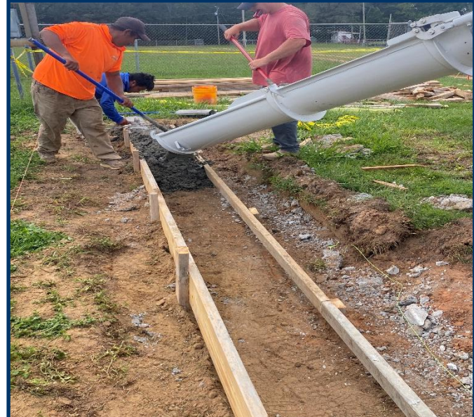
Bonifay Memorial Field Drainage Improvements Subcontractor installing NS concrete for curb and gutter in Southside Parking Area per plans.
