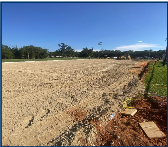
Bonifay Memorial Field Drainage Improvements Contractor installed Optional Base Material in Southside Parking Area on Veterans Blvd.
