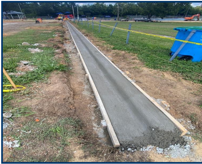
Bonifay Memorial Field Drainage Improvements Subcontractor finished curb and gutter in Southside Parking Area.
