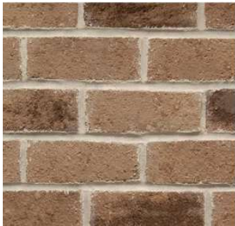
Walls / Columns Old Georgetown Material: Brick
