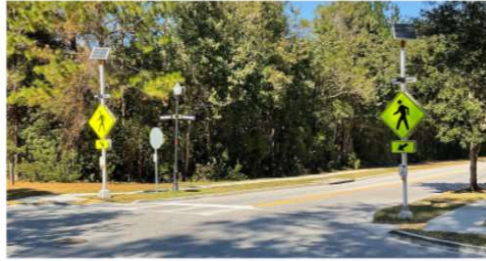
Rectangular Rapid Flashing Beacon (RRFB) Pedestrian Crosswalk
