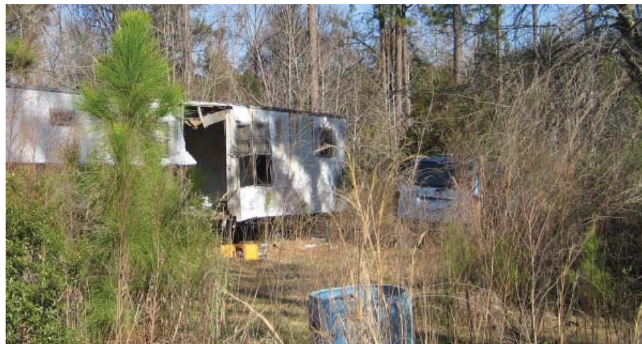
Figure 15: Overgrown lots and abandoned structures were commonly found during the community inventory.
