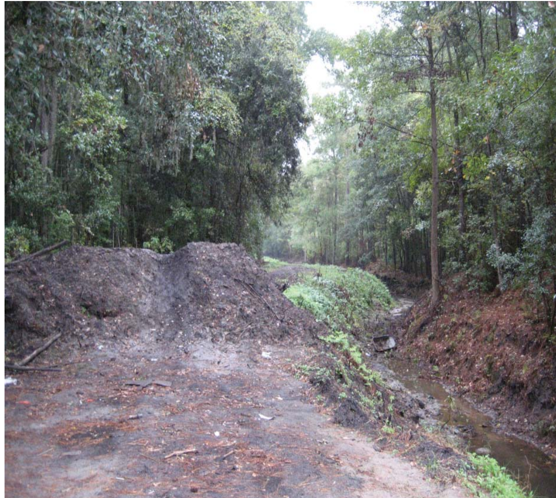
Figure 81: Primary ditch that has been cleaned out and is functioning properly.
