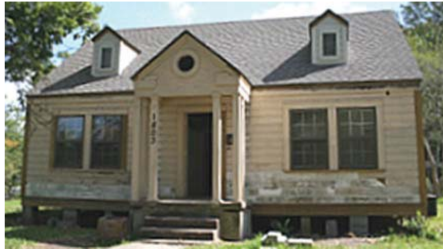
Figure 71-A: A typical house before renovation.
