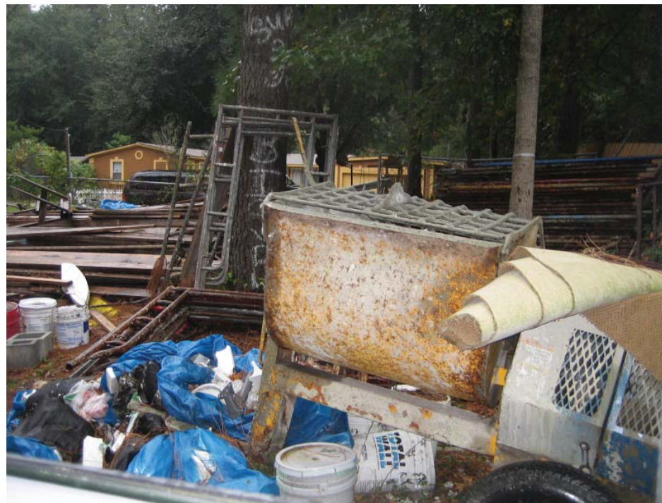
Figure 34: Stockpiled equipment and building supplies.
