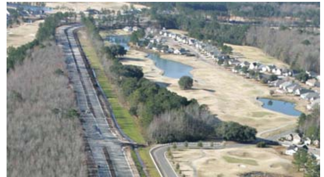
Figure 97: Existing Bluffton Parkway.
