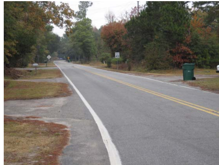
Figure 84: Buck Island Road.
