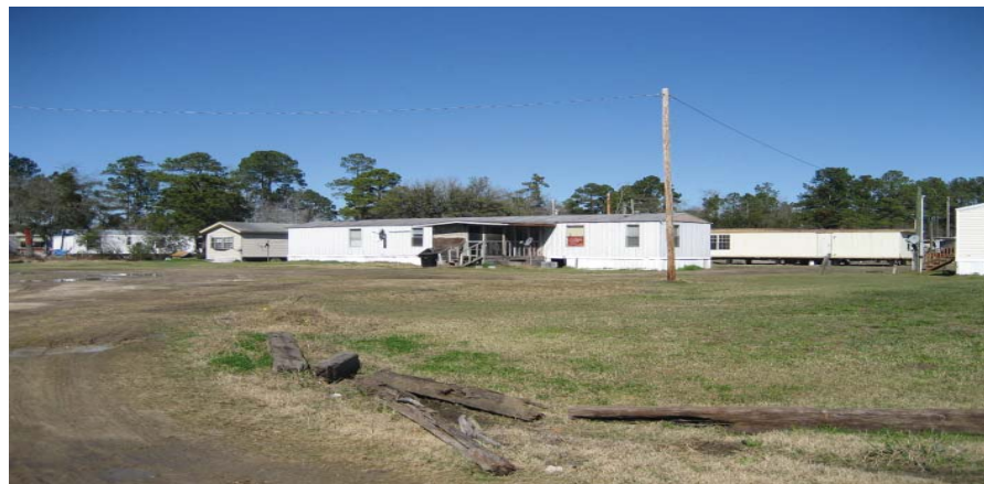
Figure 14: A manufactured home park in the BIS Neighborhood.
