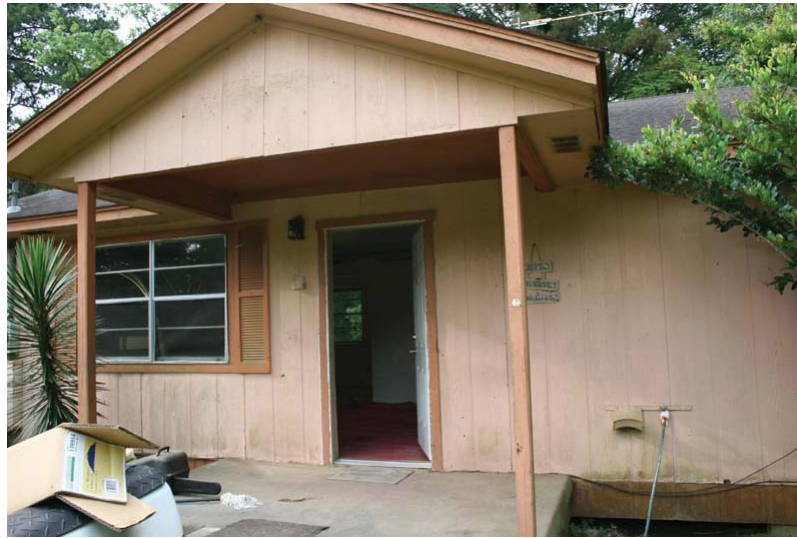
Figure 70-A: A typical house before renovation.
