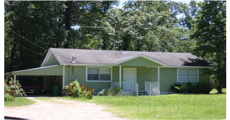
Figure 70-B: The same house after financial assistance for home repairs.
