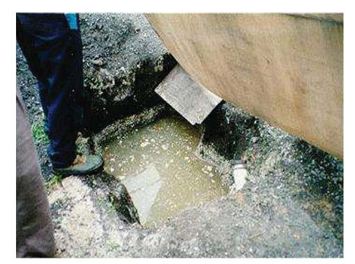
Figure 35: Failing septic tank.
