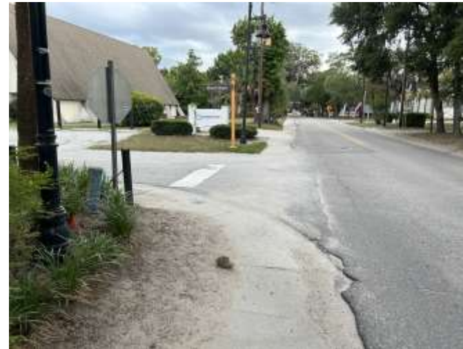
No Curb / Poor Drainage – Limited Driveway Aprons
