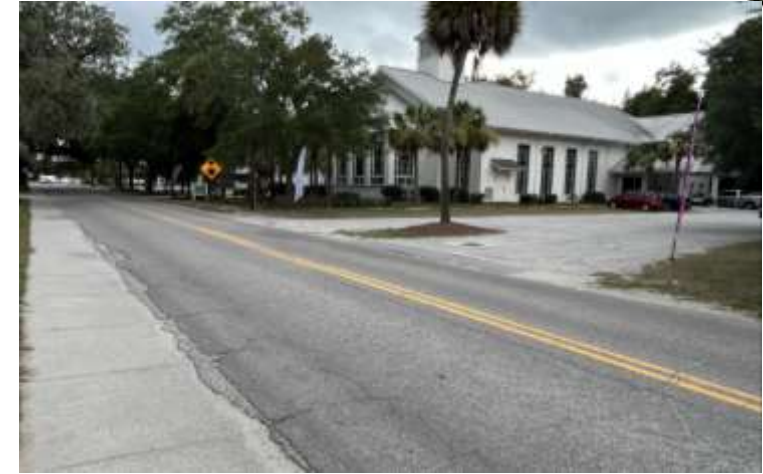
No Curb / Poor Drainage – Limited Driveway Aprons
