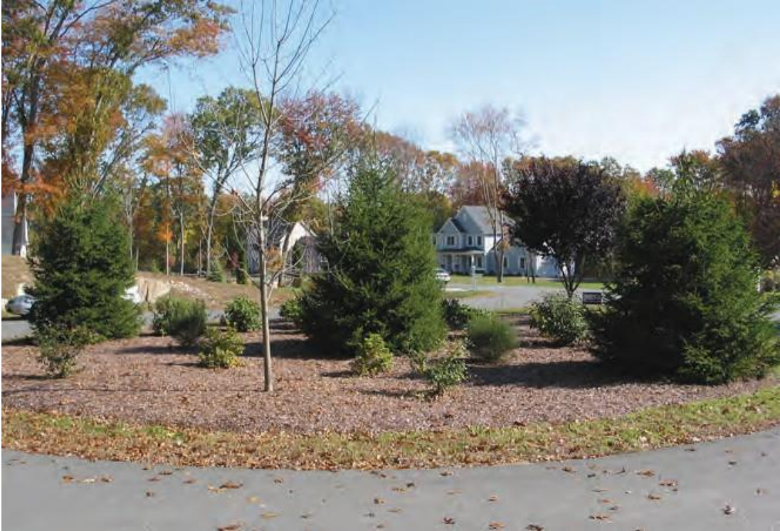
Figure 4.57. Tree Planting and Preservation in Bioretention (photo: Center for Watershed Protection)
