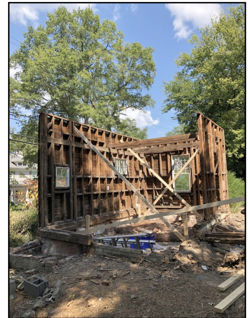
The small accessory structure above was carefully disassembled to allow for its relocation.
