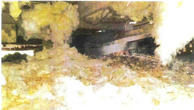
8. Crawlspace of old section (note deflected support beam)
