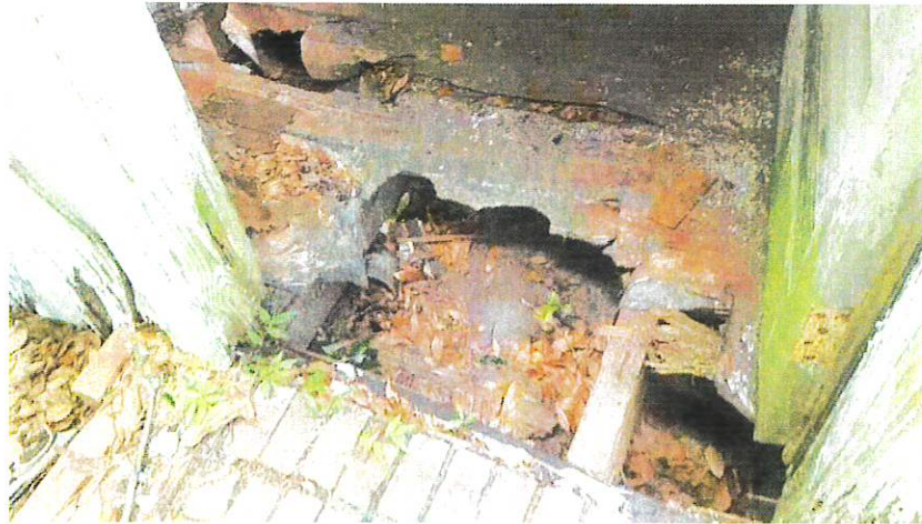
22. Deteriorated floor of BBQ shed
