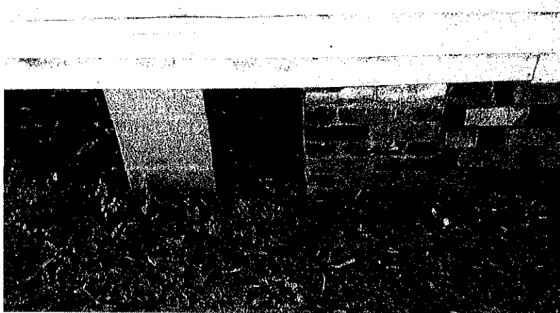
7. Foundation – Rebuilt on left; old on right
