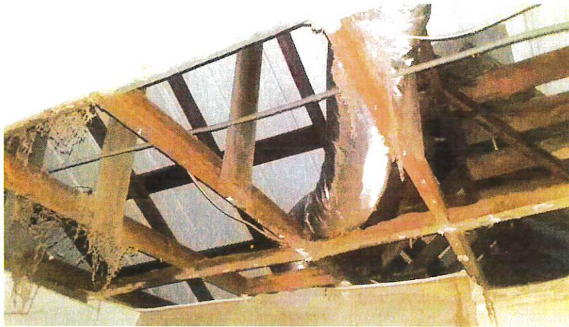
14. Ceiling collapse – old section. “Skeletal” roof structure.
