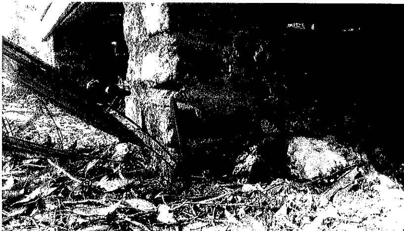
9. Brick pier of old section (mortar joint failure at base)
