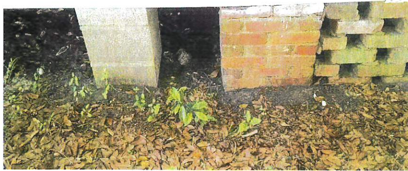
7. Foundation – Rebuilt on left; old on right
