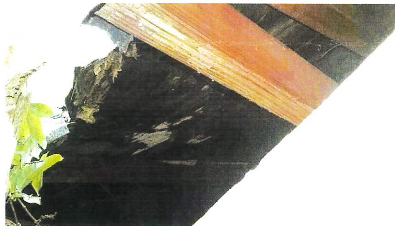
21. Deteriorated roof of BBQ shed
