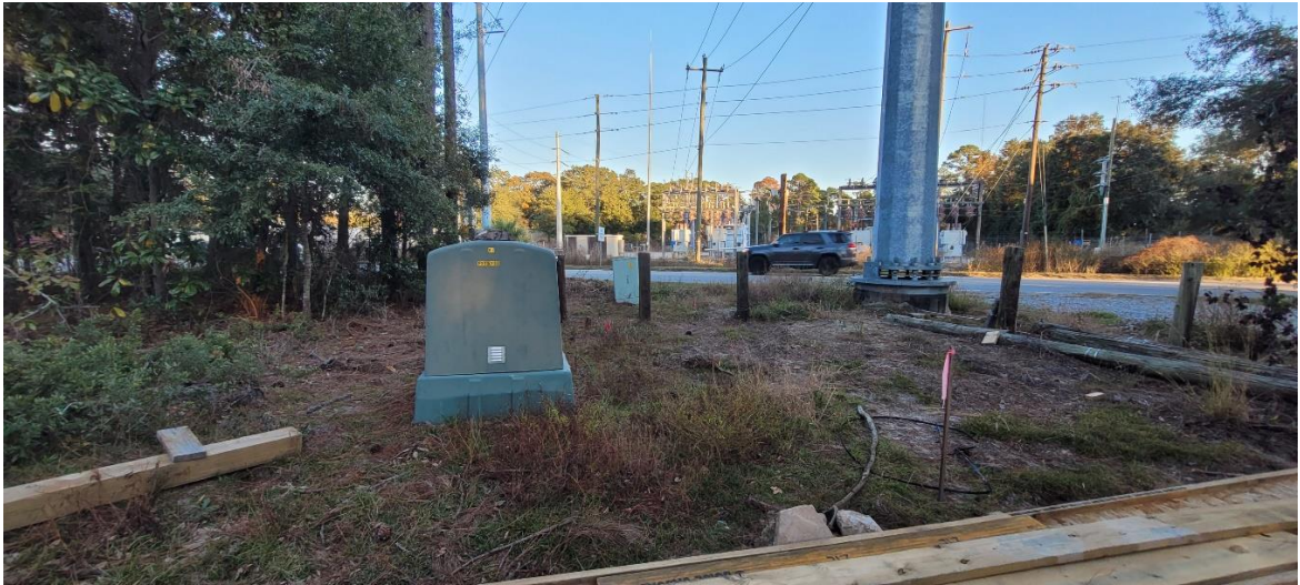
EXISTING DEAD END AT PLUFF MUD LANE
