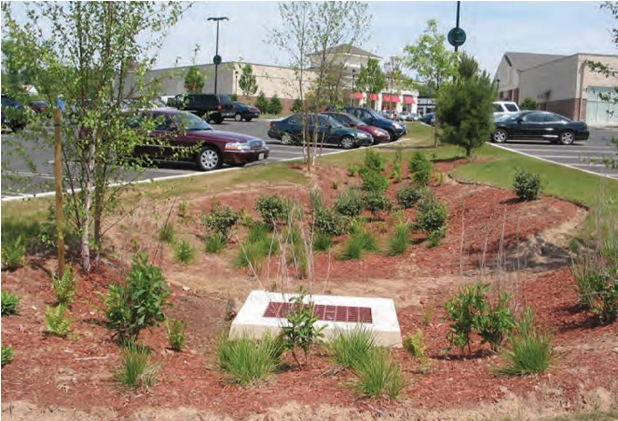
Figure 4.1. Bioretention in parking lot (photo credit: Center for Watershed Protection, Inc.).
