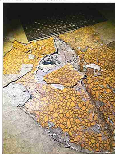
View of living room, bathroom, and kitchen ACM floor covering
