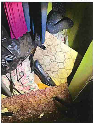
View of living room, bathroom, and kitchen ACM floor covering
