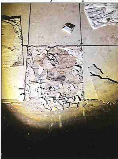
View of living room, bathroom, and kitchen ACM floor covering
