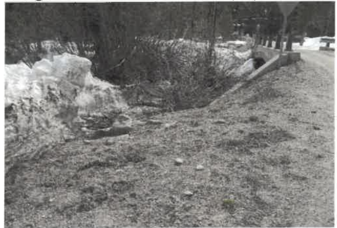
Figure 22. Damage to vegetation outside r-o-w and discharge of road base into Blue River. (May 5, 2024)
