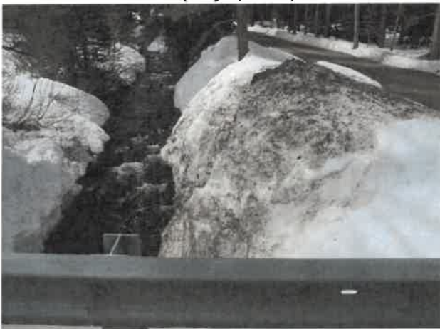
Figure 23. Discharge of road base in stacked snow bank into Blue River. (May 5, 2024)
