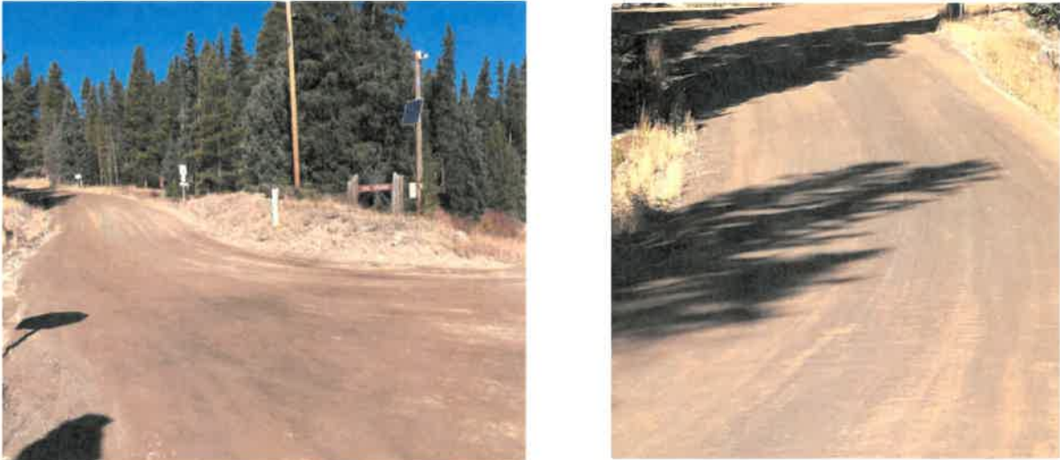
Figure 1 - Typical Surface Condition
