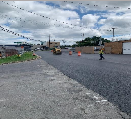
8.ADA ramps on 57 th Avenues has been completed.
