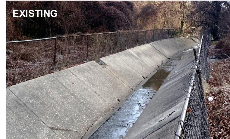
Trapezoidal Concrete Channel
