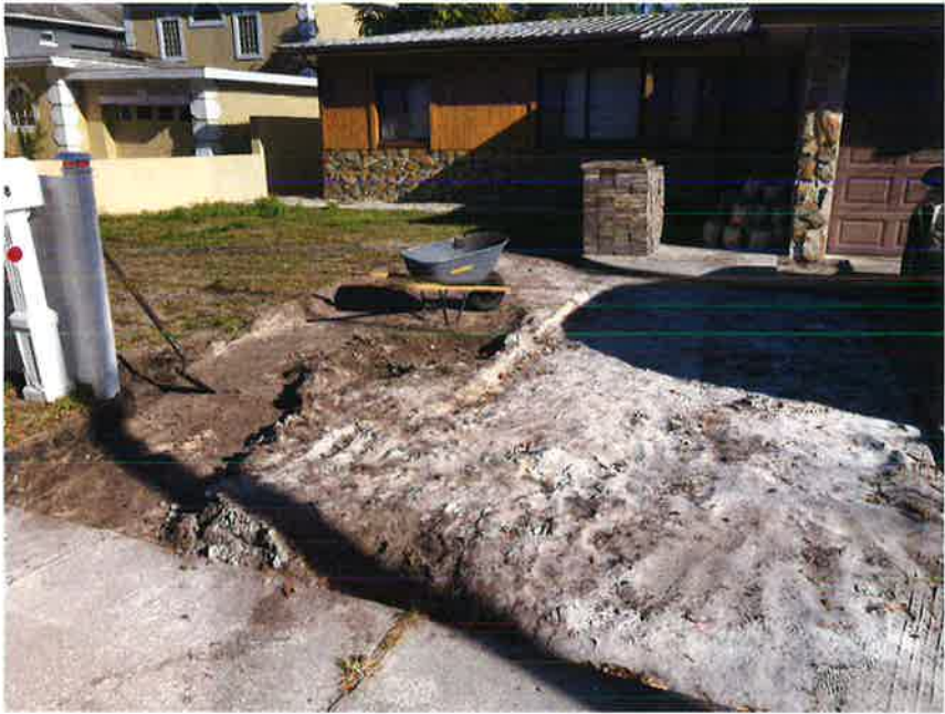
Photo 4: Example of earth sifted to a depth of 6+inches
