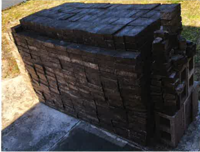
Photo 1: Paver Bricks removed to be recycled.
