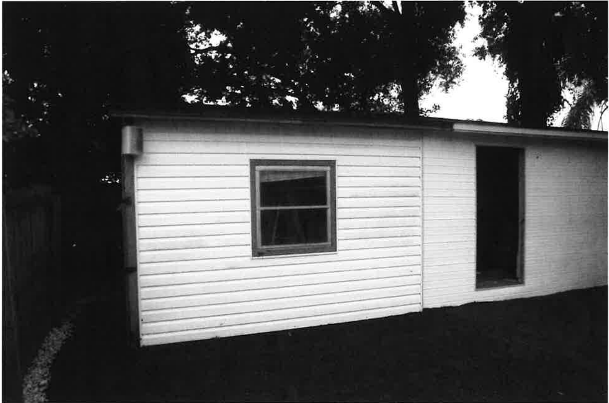
Front view of shed
