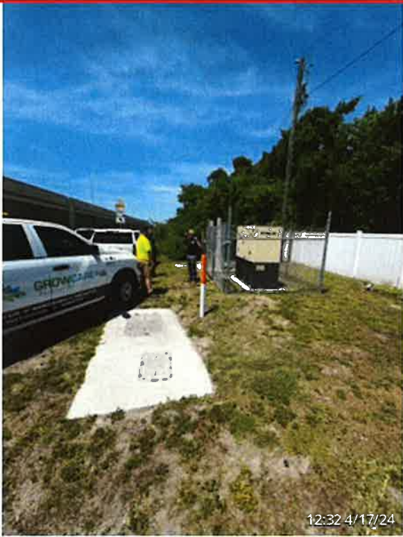
MCCOY ROW- MAINTAIN AROUND POWER BOX . . . . Corner of McCoy and Via Flora
