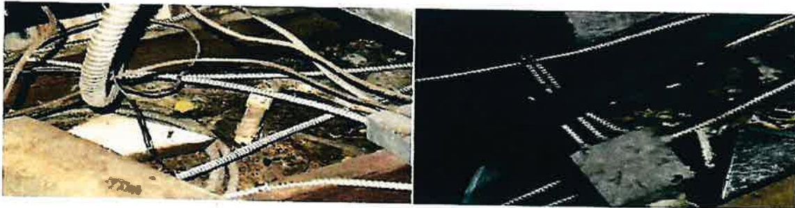
Lots of debris in the attic. Wiring is below the overflow pan. Potential electrical short if pan overflows. Insulation is torn off almost everywhere.
