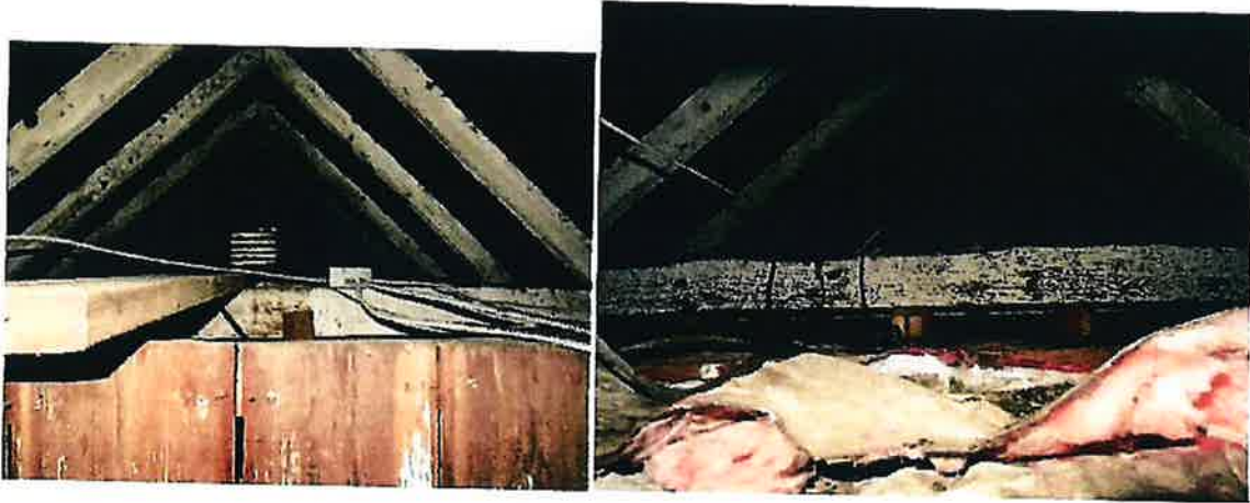
Upper attic accessed though hallway hatch. Some insulation has been laid on the ceiling, but the vapor barrier is upside down. It would have been better to have taken the vapor barrier off.
