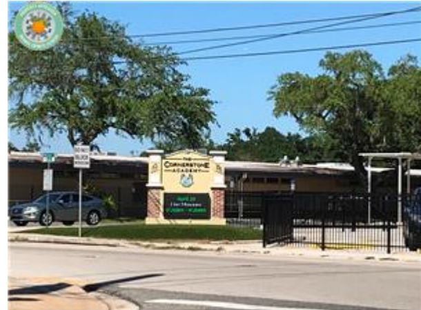
906 WALTHAM AVE, ORLANDO, FL 32809 4/16/2019 3:41 PM
