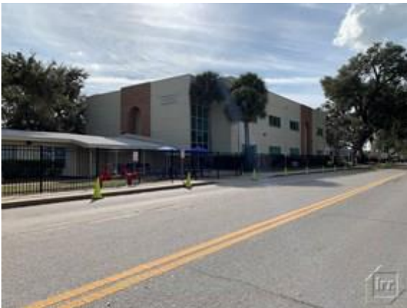
An exterior view of the elementary school. (Photograph taken on February 10, 2021)
