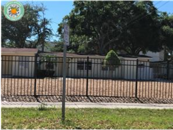
906 WALTHAM AVE, ORLANDO, FL 32809 4/16/2019 3:46 PM
