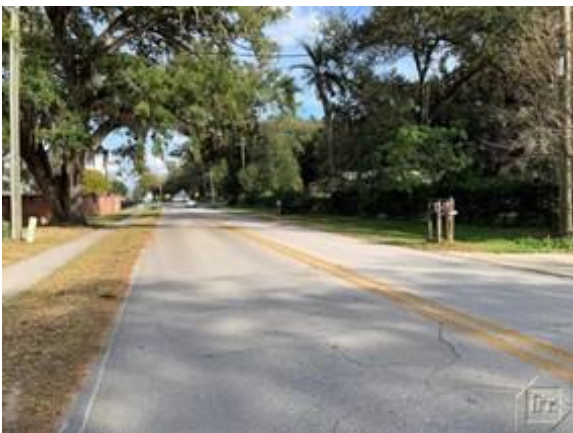
Looking west along East Wallace Street. (Photograph taken on February 10, 2021)
