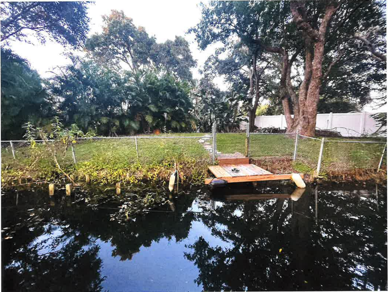
VIEW OF PROPOSED LOCATION FROM ACROSS THE CANAL
