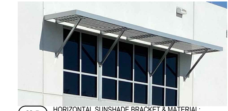
M-5 HORIZONTAL SUNSHADE BRACKET & MATERIAL: CLEAR ANODIZED ALUMINUM (SILVER)
