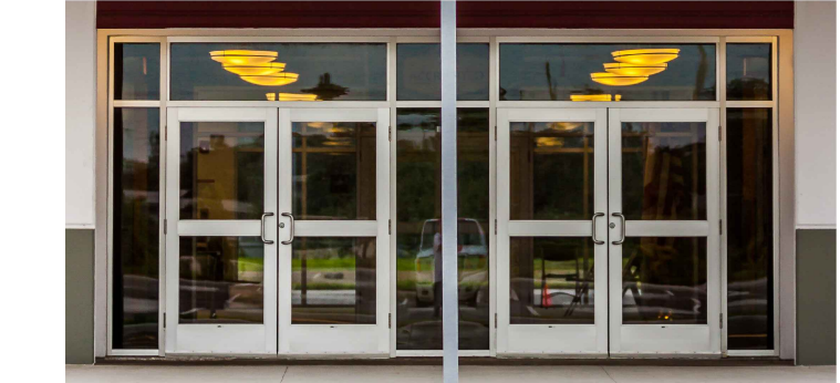
M-2 ALUM. STOREFRONTS, DOORS & WINDOWS: ANODIZED ALUMINUM W/ SOLAR-E PLUS GREY GLASS
