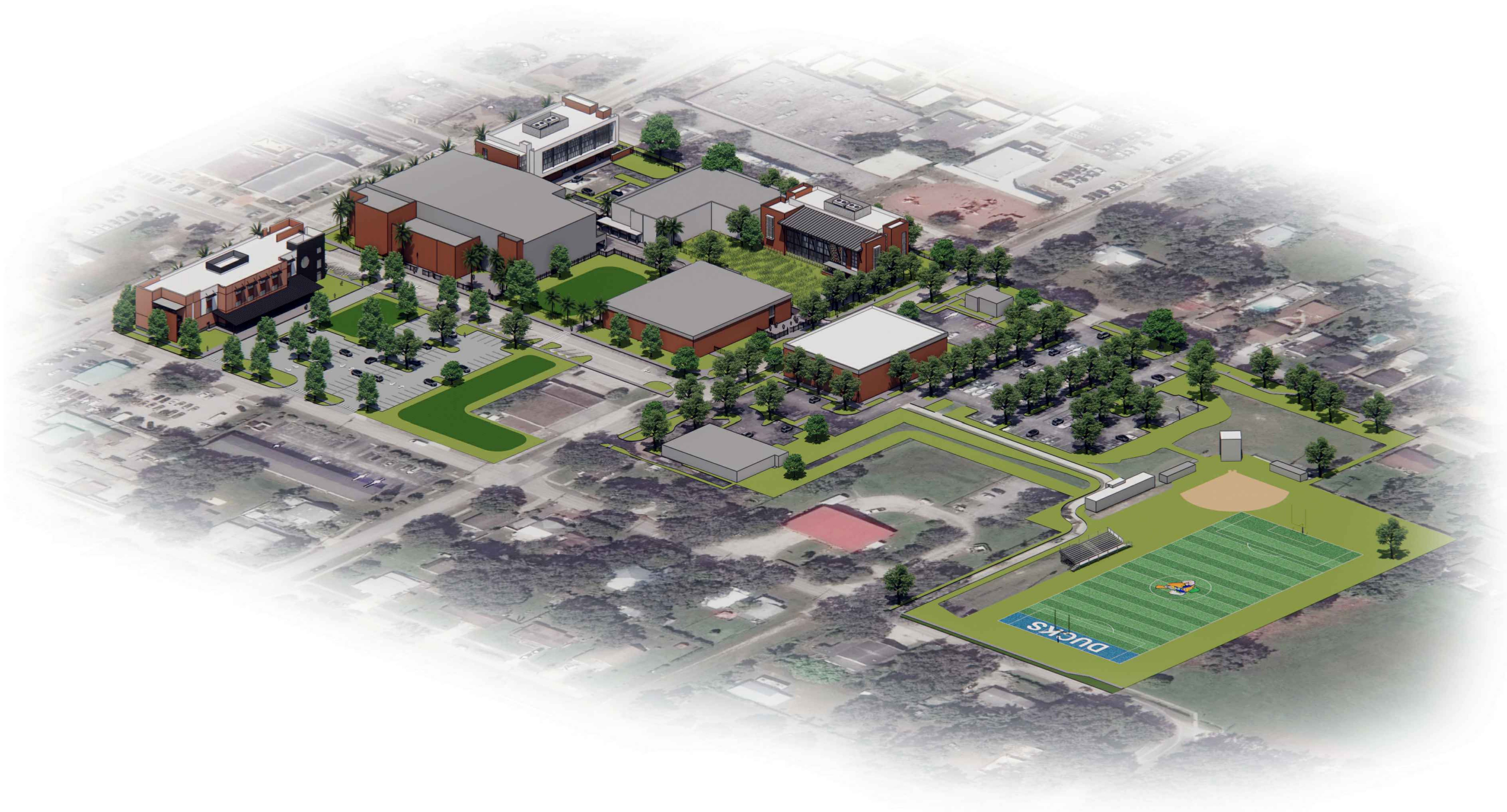
VIEW LOOKING NORTH WEST
