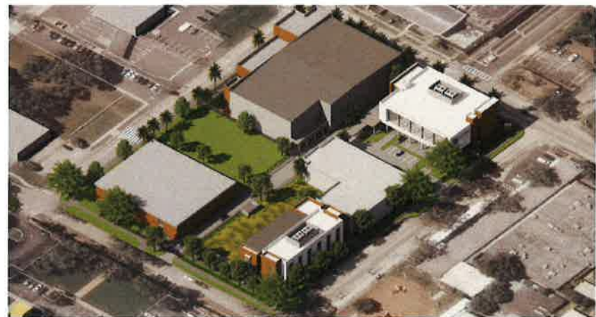
VIEW LOOKING SOUTHWEST SCALE: N.T.S. 1/2021
