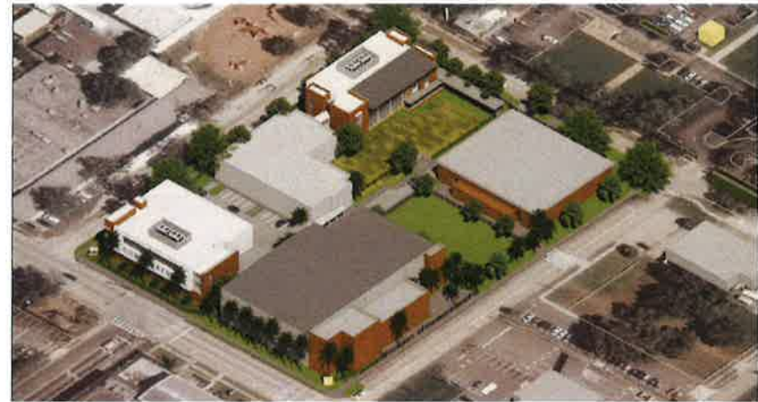
VIEW LOOKING NORTHEAST SCALE: N.T.S. 1/2021
