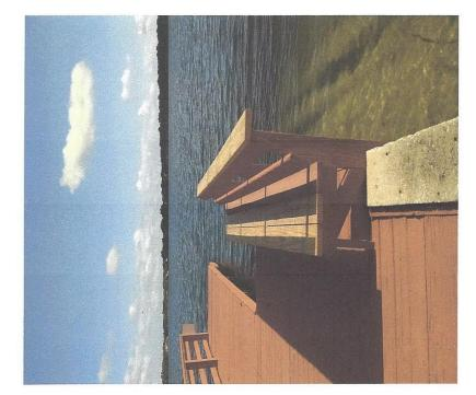
Years of weathering causing wood rot and paint checking
