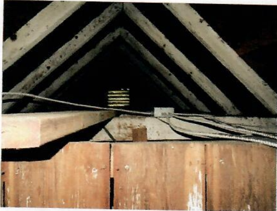
Upper attic accessed though hallway hatch. Some insulation has been laid on the ceiling, but the vapor barrier is upside down. It would have been better to have taken the vapor barrier off.
