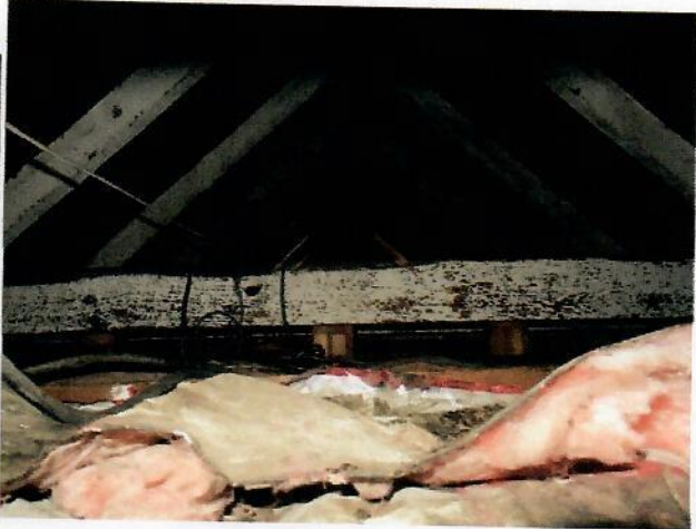
Upper attic accessed though hallway hatch. Some insulation has been laid on the ceiling, but the vapor barrier is upside down. It would have been better to have taken the vapor barrier off.
