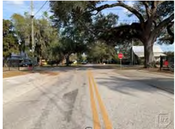
Looking east along Waltham Avenue. (Photograph taken on February 10, 2021)
