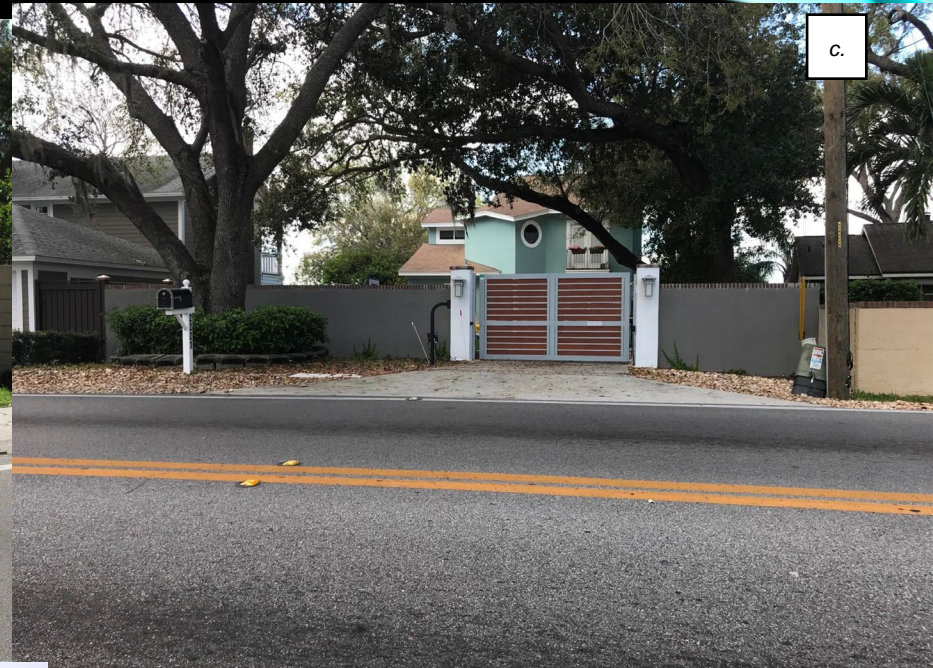
2221 HOFFNER AVE, ORLANDO, FL 32809 2/21/2018 2:20 PM
