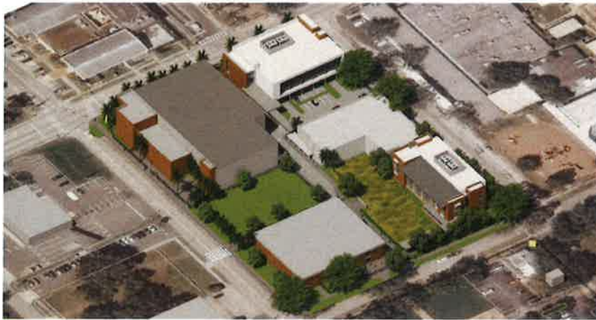
VIEW LOOKING NORTHWEST SCALE: N.T.S. 4
