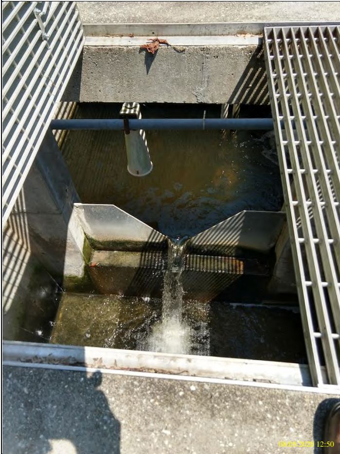
11) Final effluent sample collection point
