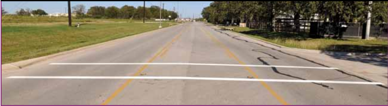
Figure 3. Photo. Example of transverse markings installed for this study.
