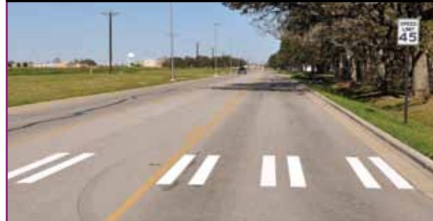
Figure 1. Photo. Example of bar pairs markings installed for this study.
