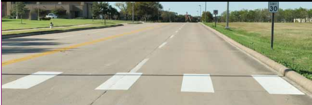
Figure 2. Photo. Example of continental markings installed for this study.
