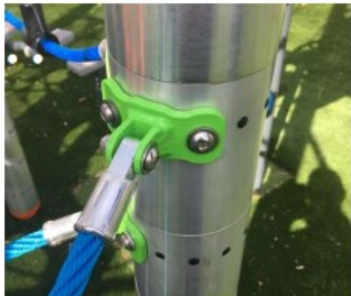
Direct bolt = shear loading at only two attachment points
