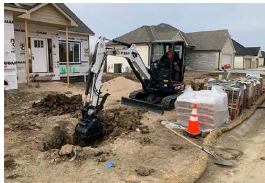
Public Works using a rented machine for precise work around fiber optic line.
