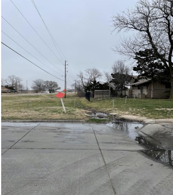
45 th and Dundee storm drain cleaning
