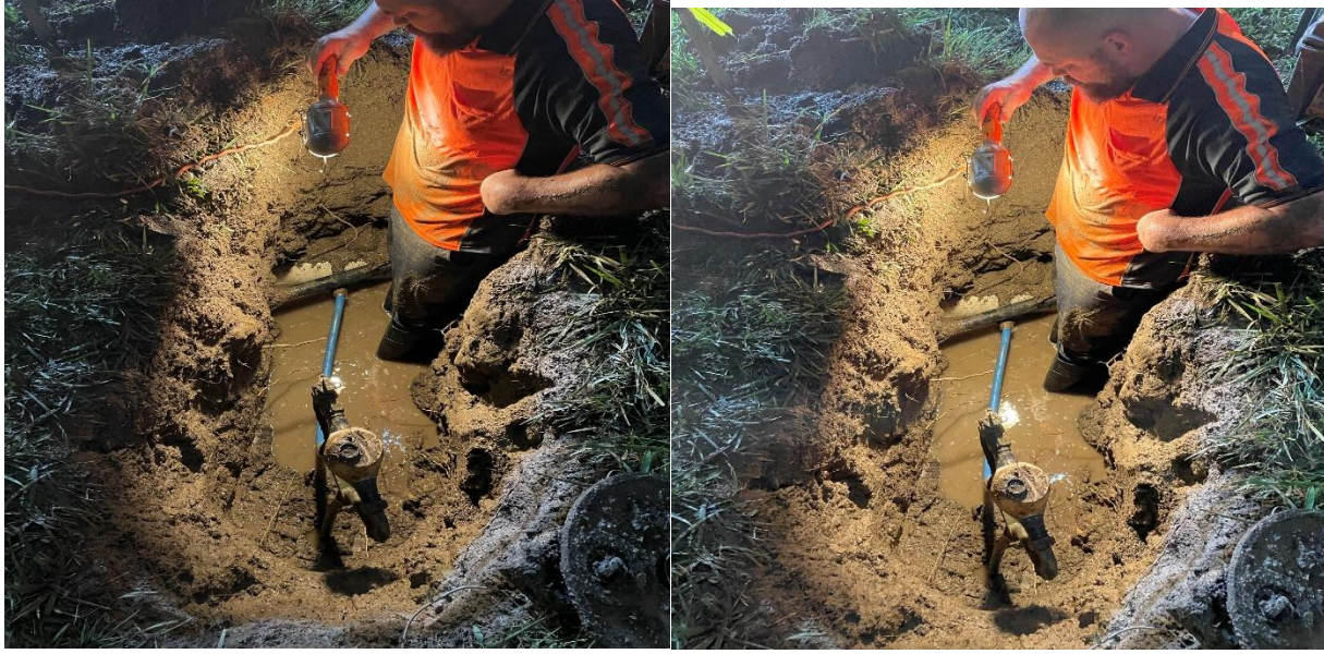
Service line repair at 5613 48 th street Circle
