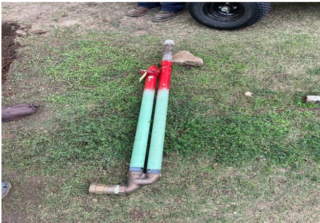
installed at Reck Center
