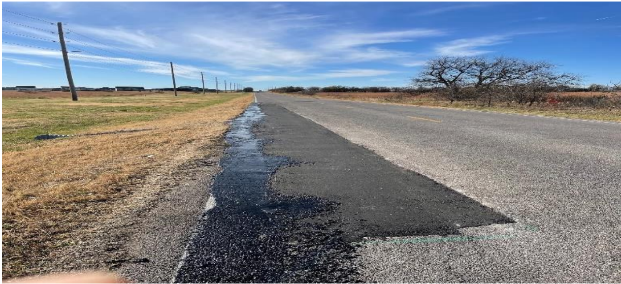
West of Rock Road on 53 rd street going West. Mastic was added for stability of the shoulder.
