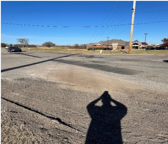
Rock Road 4-Way Stop Milled asphalt
