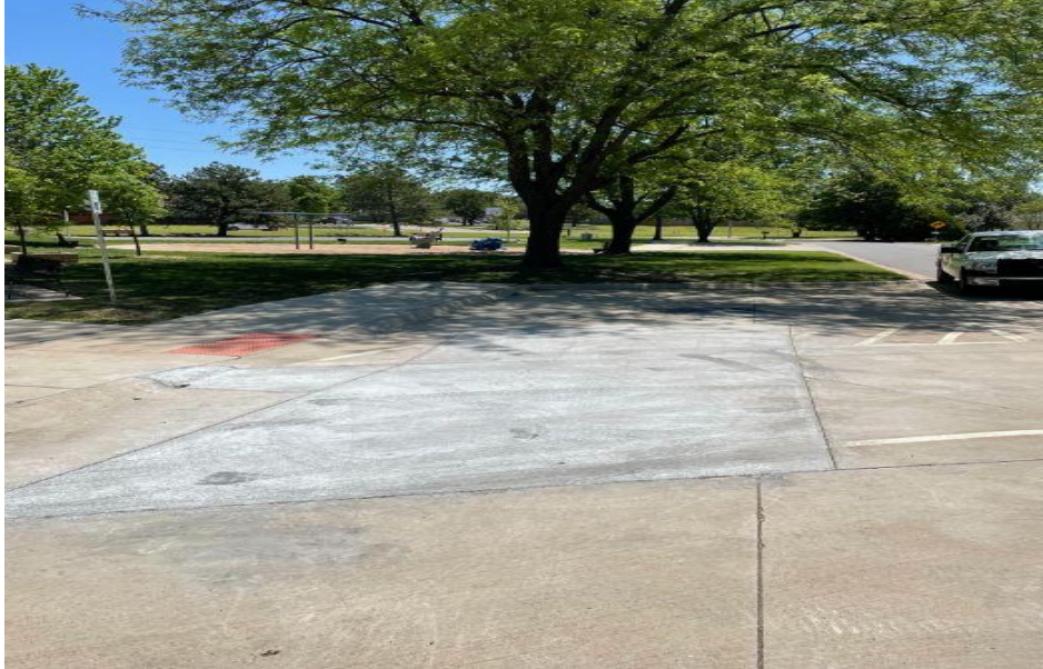
Bel Aire Park concrete repair
