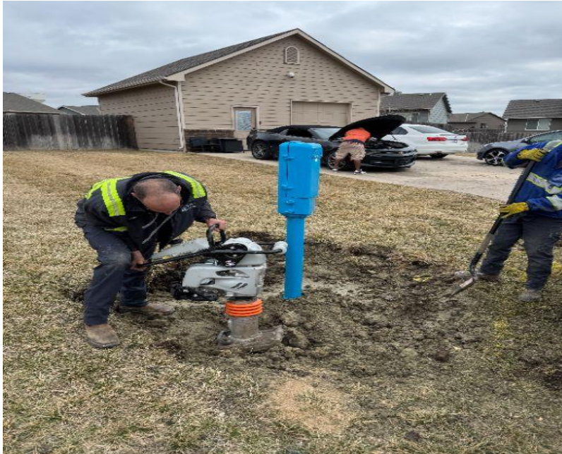
Sample Station installation
