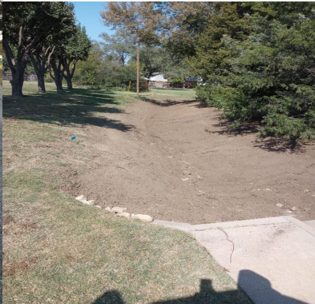
Tributary -7 regrading for drainage.
