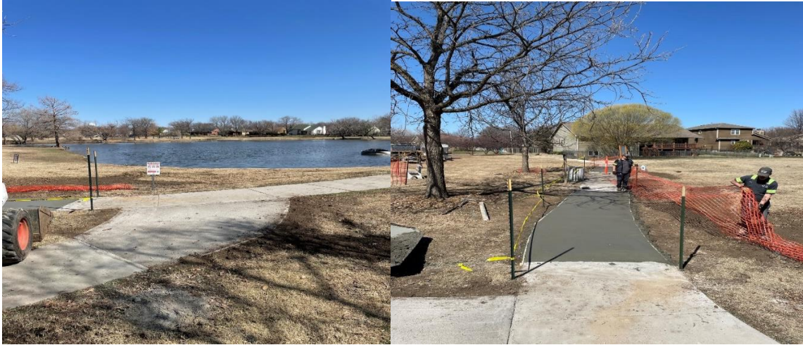
We poured several section of sidewalk at Eagle Lake.
