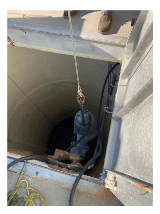
On the 25<sup>th</sup> staff received a high level alarm at the 53<sup>rd</sup> St. lift station and after inspection it was determined that the PLC (Programmable logic controller) unit failed. So the pumps were not working in automatic mode as they should. Staff had a portable pump brought in to keep the wastewater at a safe level. The new PLC was shipped overnight and replaced the next day and everything is operating as expected.
