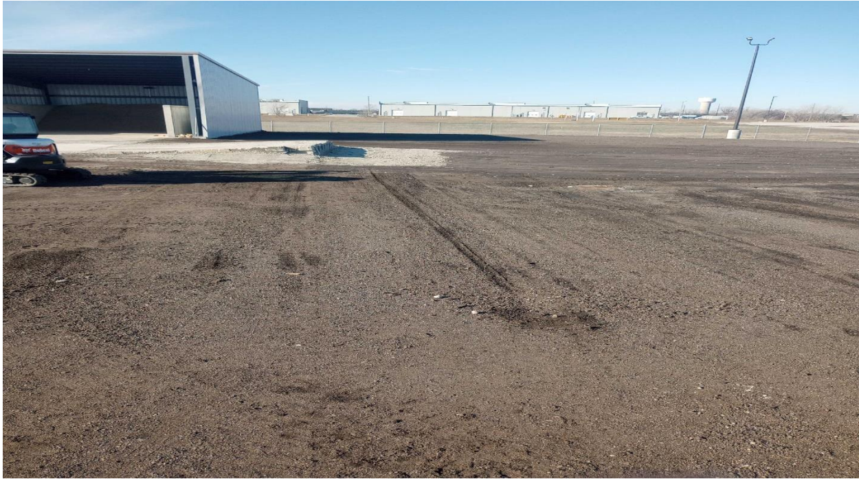
New building loading ramp for sand and salt.
