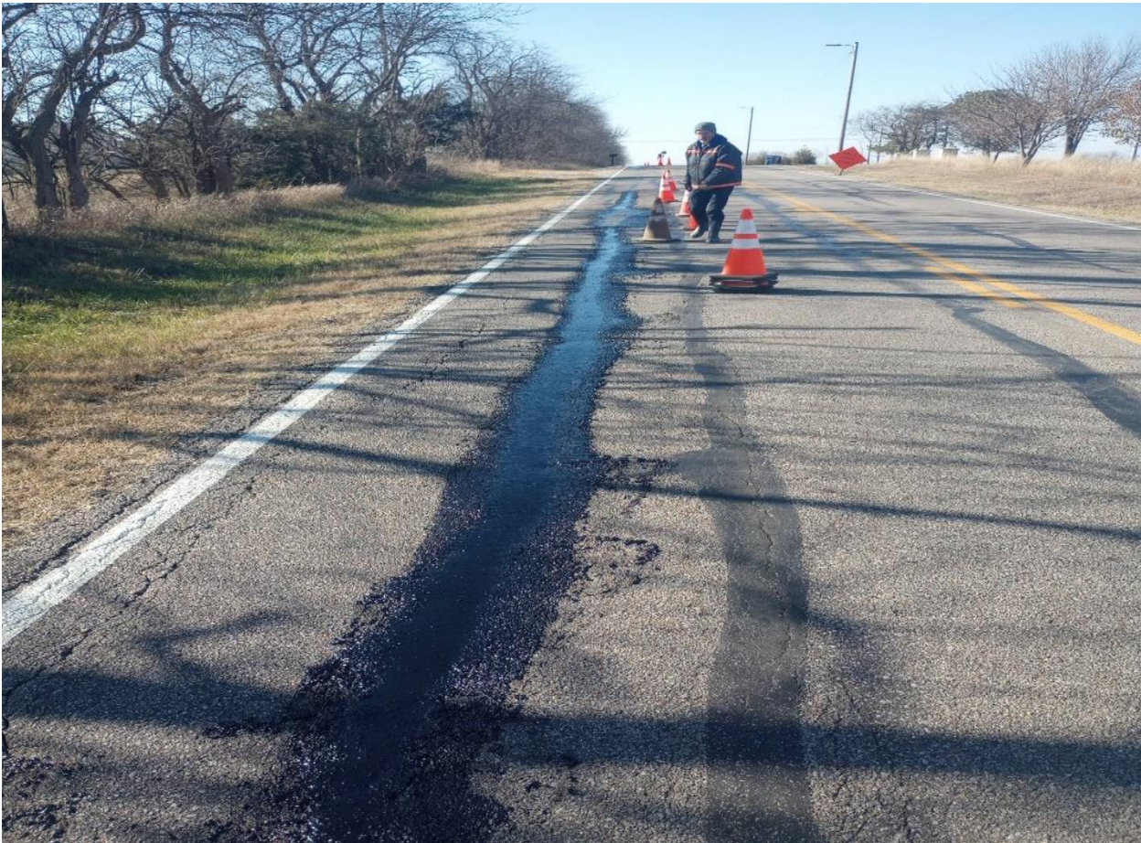
53 rd street repair
